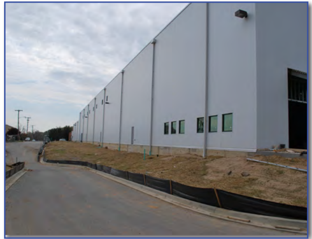
After: New Facility
