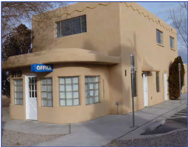
The Luna Lodge after Renovations
