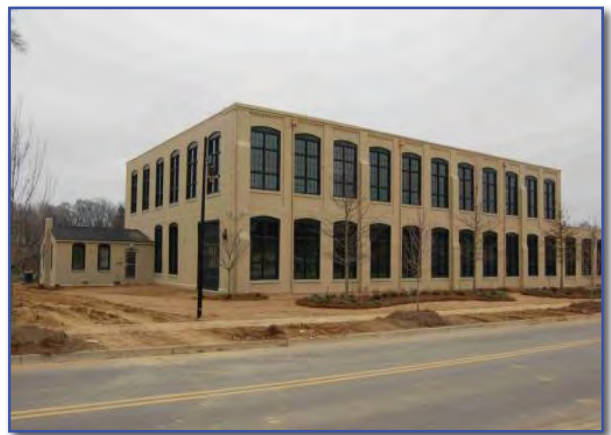
After picture of the former 1910 Building
