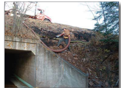
Figure 3. Applying a compost blanket on a steep, rocky slope
