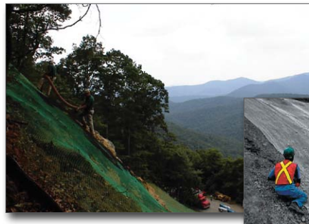
Figure 9. Netting stabilizing a compost blanket
