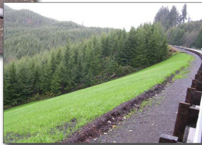
Figure 8. Using a compost berm to divert or defuse highway runoff before it reaches the compost blanket
