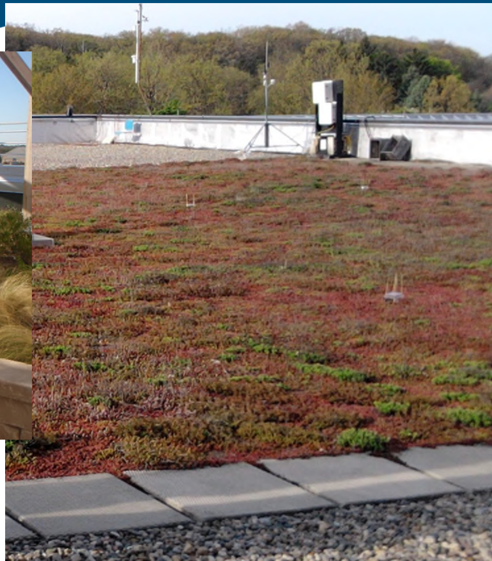
Extensive living roof
