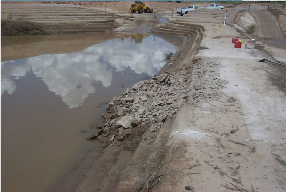
San Antonio Arroyo Sediment Basin with Retrofit Debris Containment
