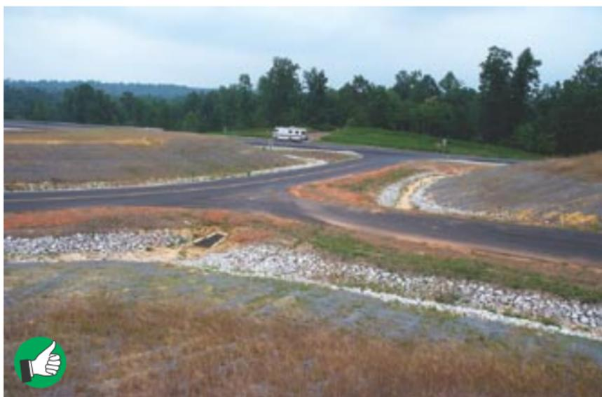
*Good construction of rip-rap lined ditches on road project. Good use of erosion blankets on slopes. Seed coverage on slopes is fair to poor.*
