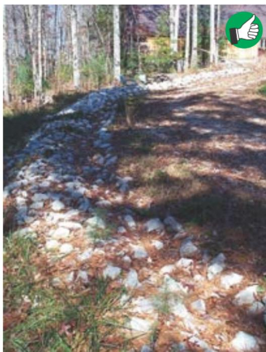
Good installation of rock-lined berm to divert rain runoff around residential construction site on steep slope near a river. Diversion ditches can be lined with grass if channel slopes are 20:1 or less, and with blankets or turf mats if they are steeper.
