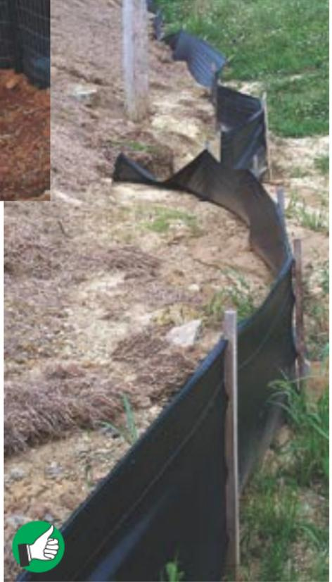
Good use of J-hook in silt fence to trap sediment in water running along fence. Sediment must be removed before it reaches halfway to top of fence.
