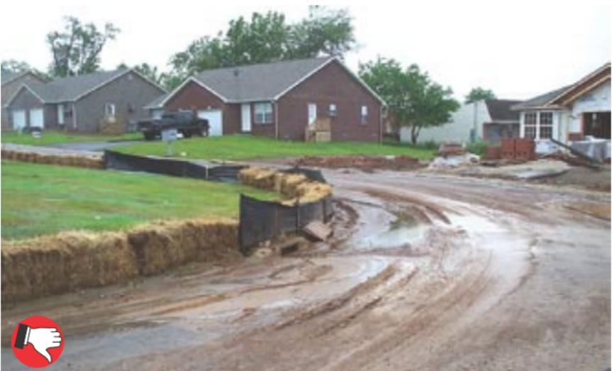
*Poor sediment filter installation, no curb inlet protection. Bales alone provide poor protection (note mud on pavement). Very good seed application.*
