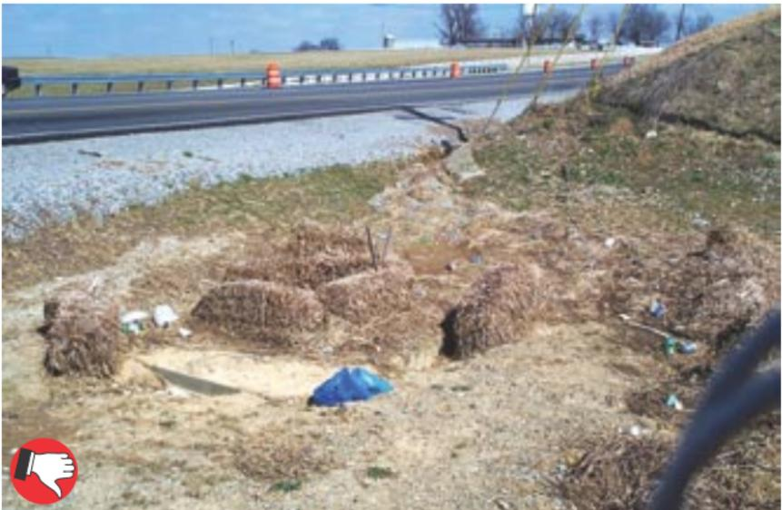
Poor protection for drop inlet on concrete pad. Straw bales make good mulch but are not suited for inlet protection or silt check dams.
