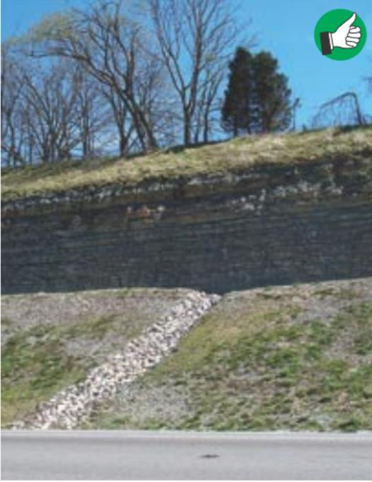
Very good application of rock lined down drain channel to carry water down slope face. Use filter fabric under rock. Install multiple drains at appropriate spacing where flows are heavy. Install flow dissipaters at outlet to absorb energy of the discharge.
