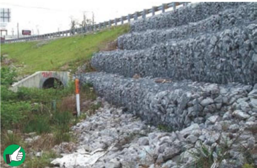
Good use of rock-filled, stacked gabion baskets to protect steep slope. Soil and bark mulch can be used in or over gabions and planted with live willow or hardwood cuttings to reduce "hardened" look.
