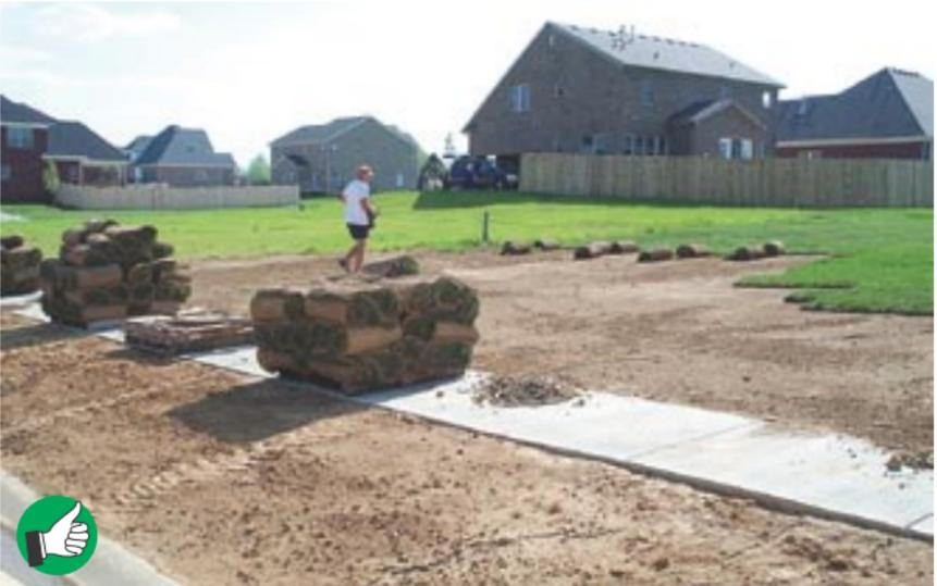
*Installing sod immediately after grading work is complete can reduce erosion and sediment loss to near zero.*
