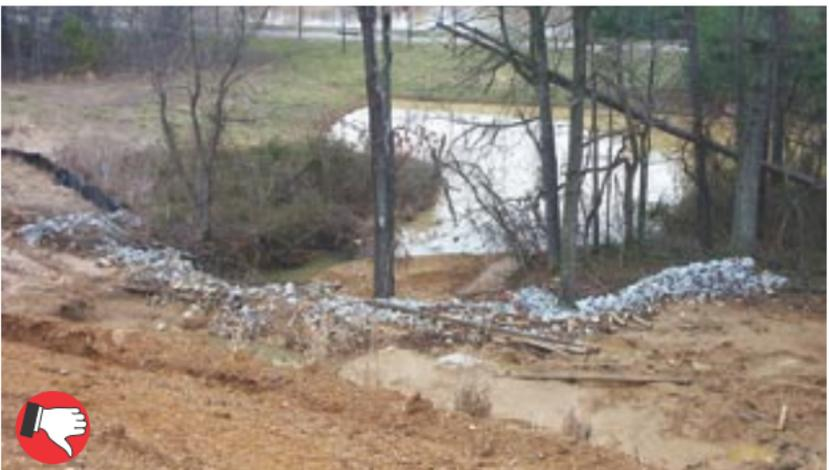
Poor sediment trap construction. Dike is poorly built, without an overflow notch. Placement is too close to pond. No seeding or mulching evident in drainage area.
