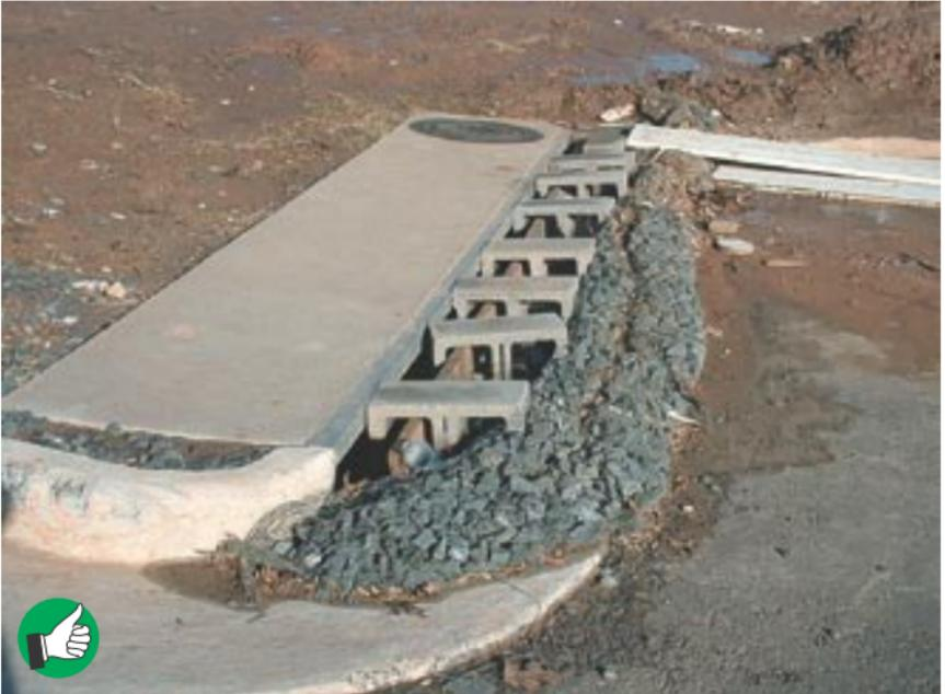
*Excellent use of concrete blocks and #57 rock for ponding dam to protect inlet. Note 2"x 4" board through blocks for stabilization. Note galvanized fencing and filter fabric between block and rocks.*
