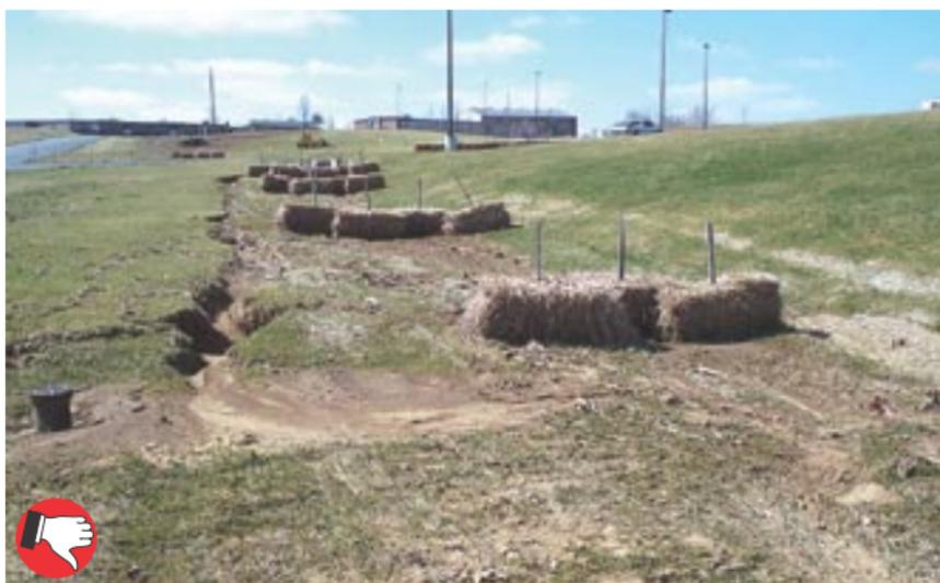
Poor silt check installation. Straw bales are not approved as silt checks for ditch or channel applications due to rotting, installation difficulties, and high failure potential.
