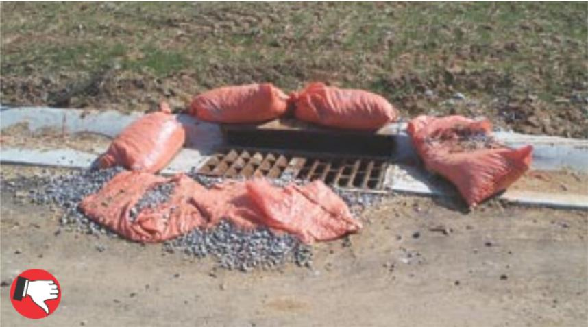
Poor placement of stone bag inlet dam; poor education of construction site drivers. Bags work well if used properly and maintained. Bags must form a dam around the inlet with no large gaps.
