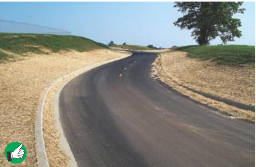
*Very good treatment of roadside areas with blown straw after seeding. In areas near lakes, streams, and rivers, straw in roadway must be cleaned up after application.*
