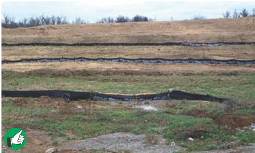
*Very good installation of multiple silt fences on long slope. Turn ends of fencing uphill to prevent bypass. Leave silt fences up until grass is well established on all areas of the slope. Re-seed bare areas as soon as possible. Remove or spread accumulated sediment and remove silt fence after all grass is up.*
