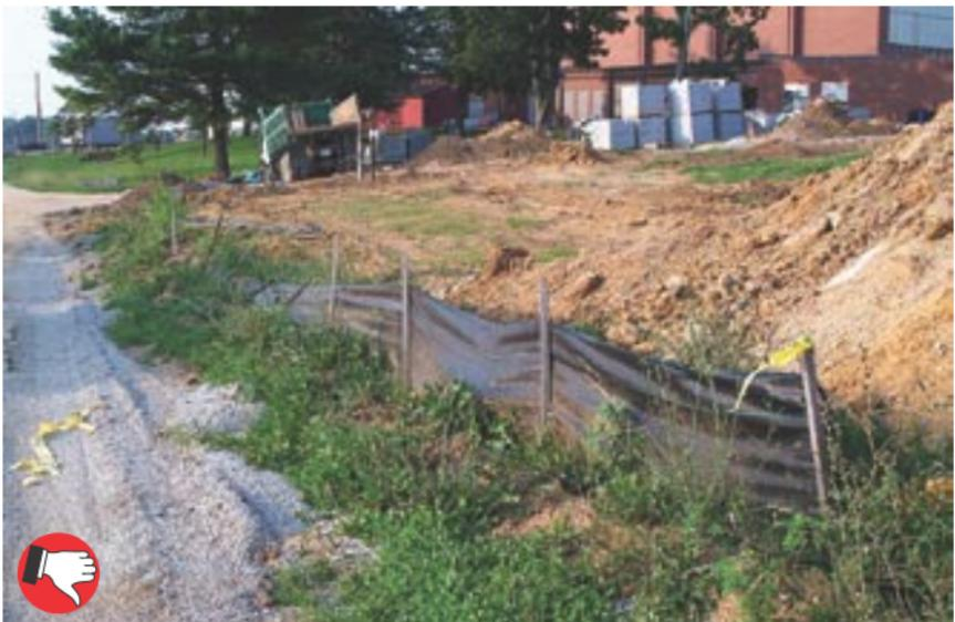
*Very poor attention to silt fence maintenance. Fences and other sediment controls must be inspected and repaired weekly; activities should be logged.*
