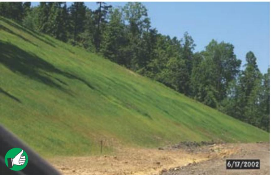
Excellent slope protection with seeding and erosion control blanket. Blankets or mats are required on most projects if slopes are 3:1 or steeper. KYTC requires blankets on all slopes longer than 100 feet if they are 4:1 or steeper.
