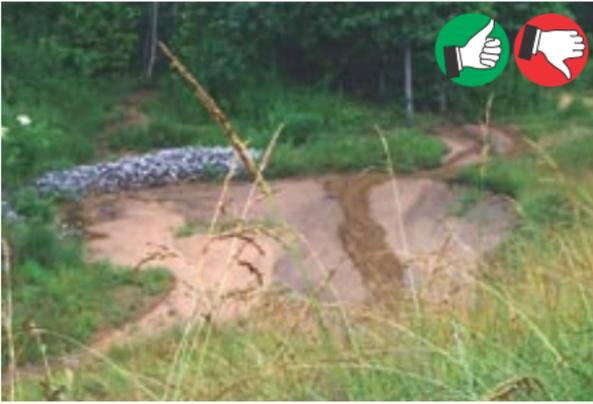
Good sediment trap installation, but poor maintenance has caused trap to fill and bypass to occur. Remove sediment before trap is half full. Make sure containment dike has an overflow notch to control the discharge location.
