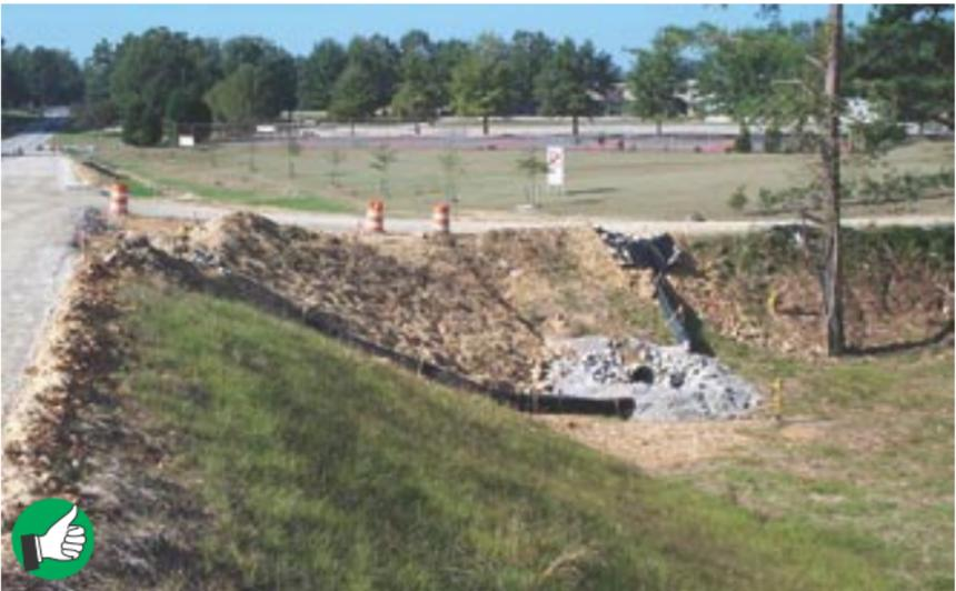
Very good use of 20-inch plastic slope drain pipes to convey water from roadway to lower channel. Note staking and rock anchoring at bottom of temporary slope drain pipes.
