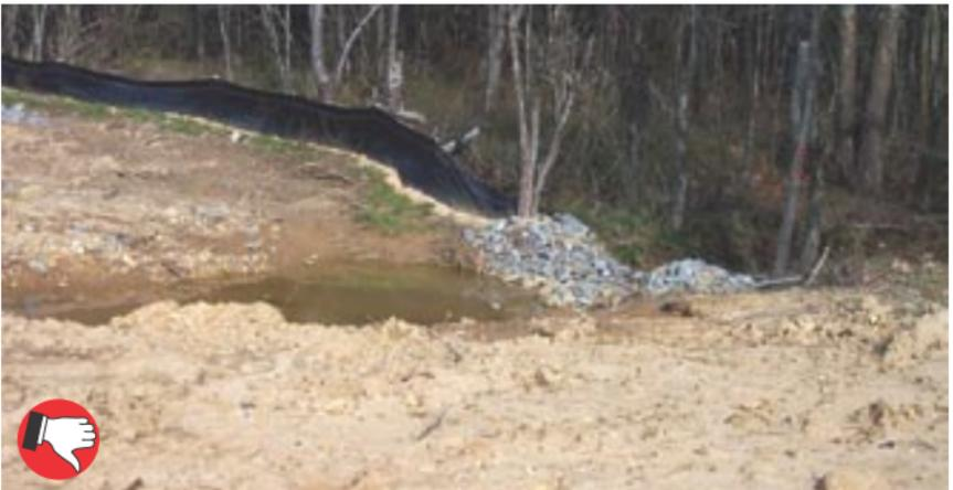
Fair to poor trap installation. Dike overflow notch is too deep; basin is too small. No seed or mulch covering bare soil areas.
