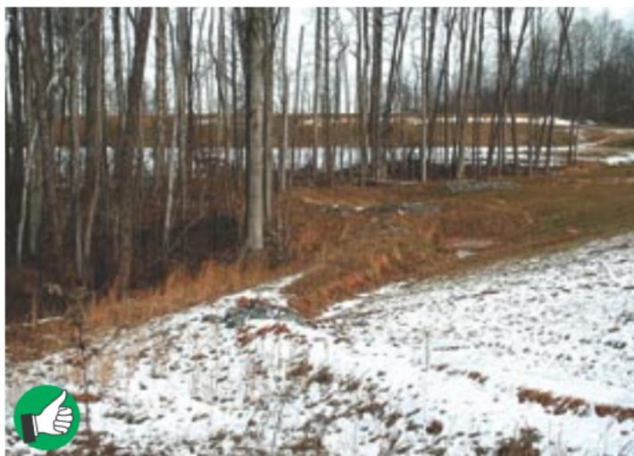
Well built vegetated berm diverting runoff from wooded stream. Diversion berms and ditches should be seeded after construction. Use blankets if slopes are steep.
