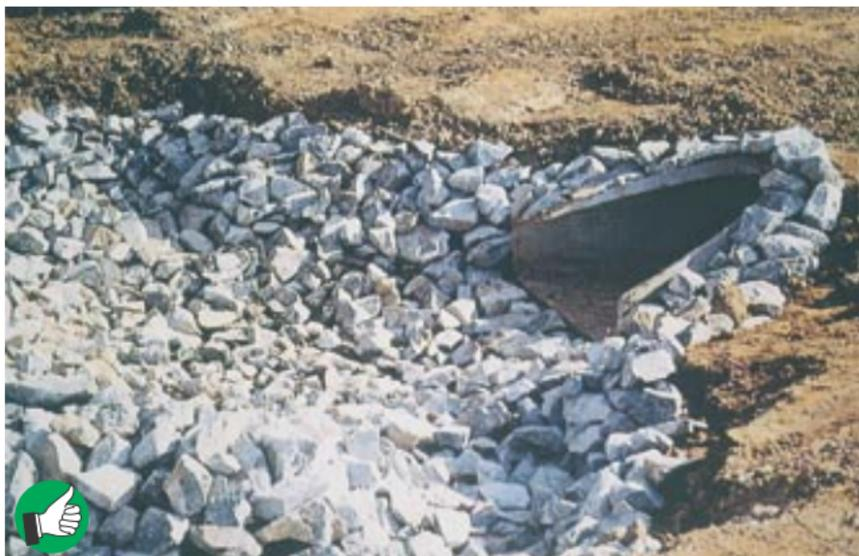
Excellent placement and construction of rock apron to dissipate flows from culvert outlet. Area needs seeding and mulching.
