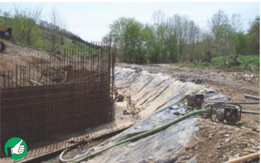
Excellent use of temporary plastic covering during bridge construction to reduce slope erosion. Filter sediment from pump discharges or discharge to protected infiltration area away from waterways.
