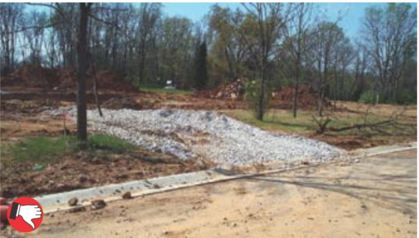
Rock pad was installed properly with right sized rock, but lack of filter fabric underliner is causing rock to spread and sink into the soil. Note tracking of mud onto paved road. Mud tracked on roadways violates BMP standards, and is a potential legal liability.
