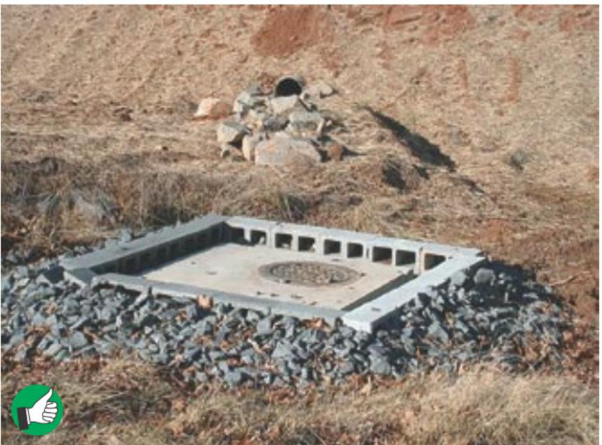
*Very good design and installation of inlet protection ponding dam using concrete blocks and rock. Outlet pipe in background has a rock apron to dissipate flows.*
