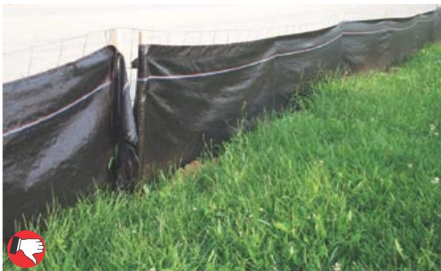
*Poor installation where silt fences are joined. Roll end stakes together before driving in to create an unbroken sediment barrier or lap curved sections to prevent bypasses. Leaving grass strip between silt fence and bare soil area is a good idea.*
