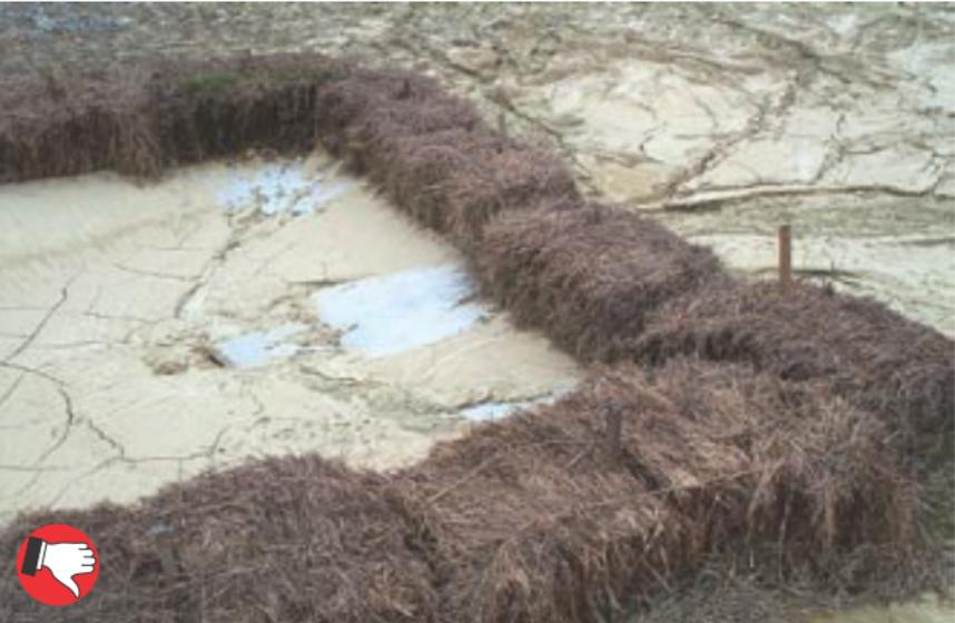
Straw bales have rotted and failed, with muddy runoff undercutting bales. Concrete apron and drop inlet grate are nearly covered in sediment. Use straw for mulch only.
