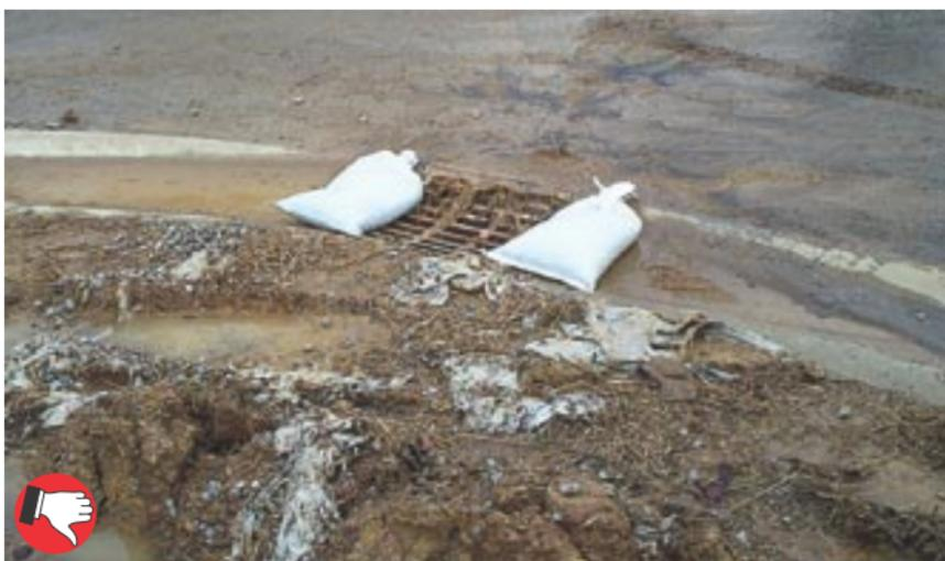
*Poor job of seeding and protecting curb inlet with stone bags. Project should not be closed out until all bare soil areas are vegetated and all temporary controls (inlet dams, silt checks, silt fencing) have been removed. File “Notice of Termination” with the KY Division of Water when project is completed.*
