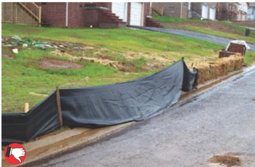
*Poor installation of silt fencing, fair to good seeding. Silt fence must be trenched in along bottom. Straw bales are not approved as sediment barriers.*
