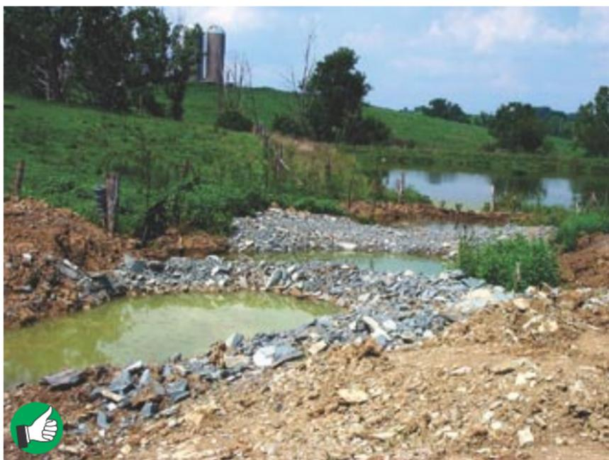
*Fair installation of two traps above small pond. Dikes are a little too small; placement is too close to pond. Area needs seed and mulch.*
