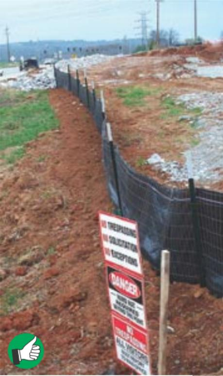
Very good use of continuous “super” (reinforced) silt fence and shot rock sediment barrier (far side) to filter muddy runoff from commercial development site. Note that wire fencing is installed between the filter fabric and the posts.
