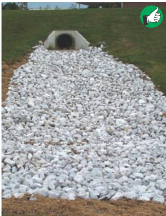
Good placement and construction of rock apron at high-flow culvert outlet. If flow from culvert enters a channel, make sure channel is lined with grass, and blankets or mats, if necessary, to prevent erosion.
