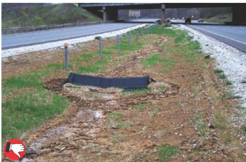
Poor application of commercial silt check product. Check dam needs to be longer (tied into banks). More are needed, at correct spacing for channel slope. Area needs to be re-seeded; ditch may need blanket liner.
