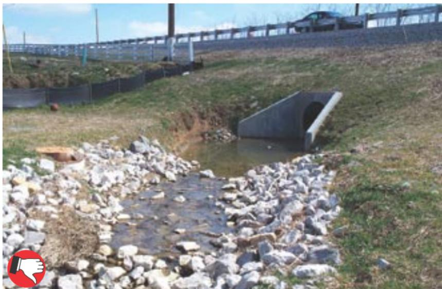
Good silt fence installation, fair seeding and mulching on slopes. Poor placement and construction of flow dissipater apron at culvert outlet.
