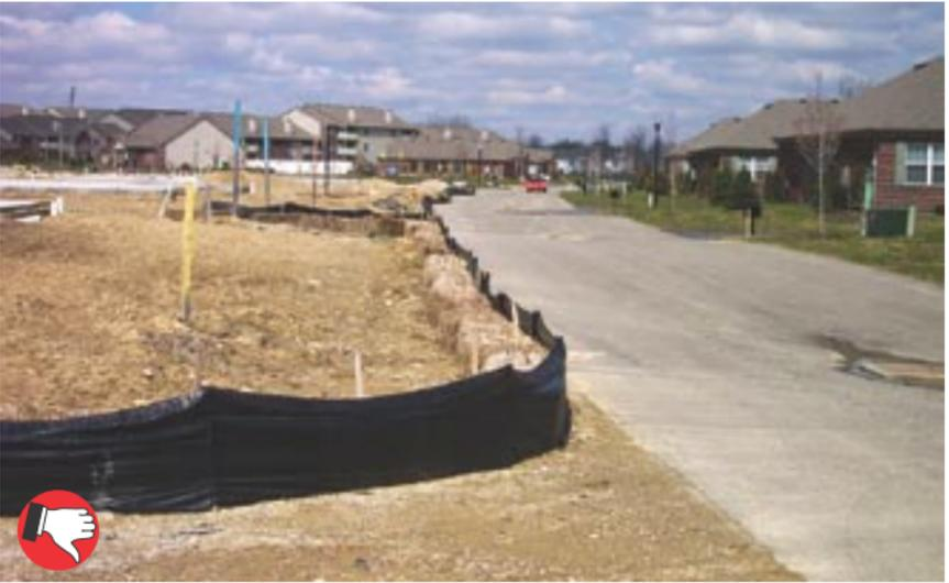
*Sediment barrier installed backwards. Silt fence fabric should face bare soil area. Stakes go on downhill side. Straw bales can be used to back up fence on downhill side, but not alone.*
