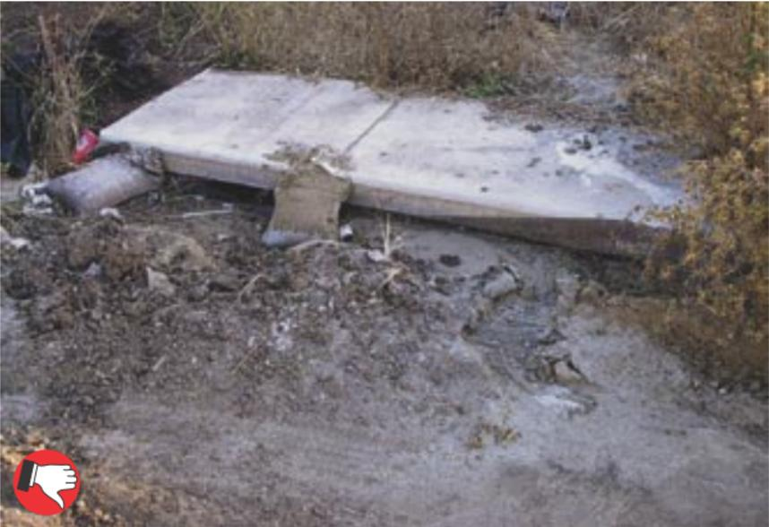
Poor placement and poor maintenance of stone bag inlet ponding dam. Accumulated sediment must be removed and dam should be repaired after each half-inch rain.
