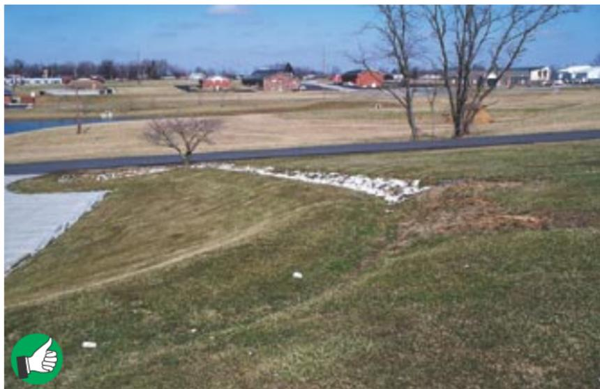
Good construction, seeding, and stabilization of diversion berm. Note that diversion ditch is lined with grass on flatter part of slope, and with rock on steeper part.
