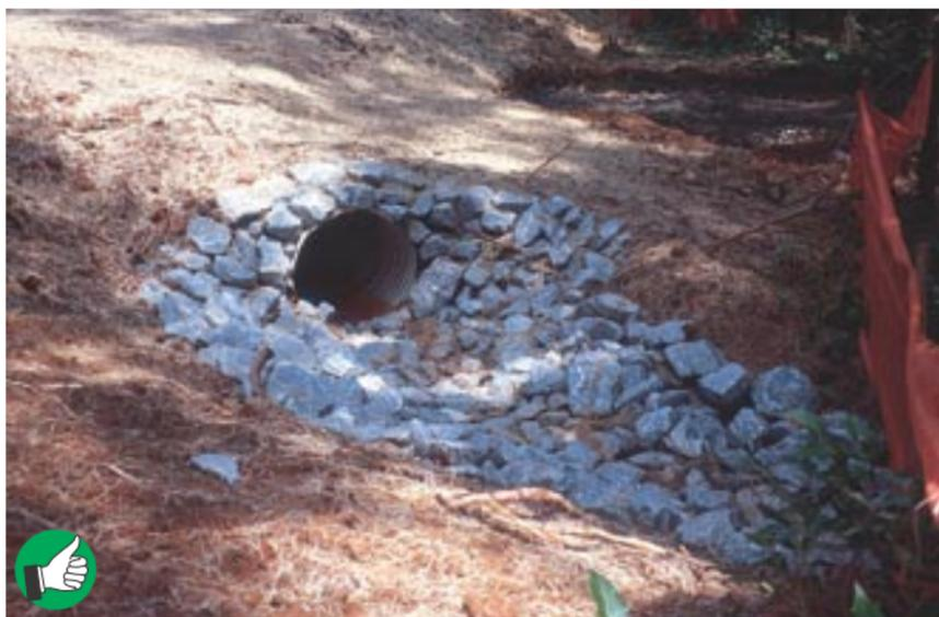
*Excellent installation of rock flow dissipater at culvert outlet. Make sure inlets, outlets, and slopes are well stabilized before leaving the site and filing your “Notice of Termination” for ending permit coverage.*
