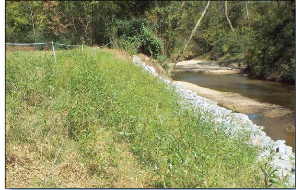
Figure 3. This riparian buffer and streambank stabilization project protects Hog Creek.
