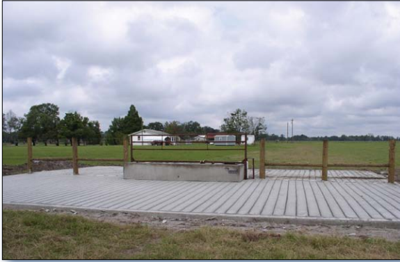
Figure 2. This farmer combined heavy use area protection with an alternate watering source.
