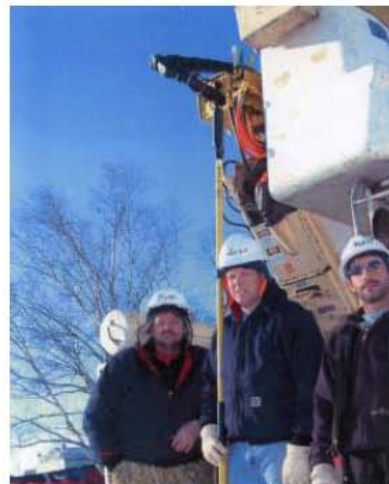
PCB transformer phase-out (Grand Marais, MN)
