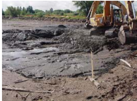
Close-up view of the contaminated sediments being removed from Hog Island Inlet.
