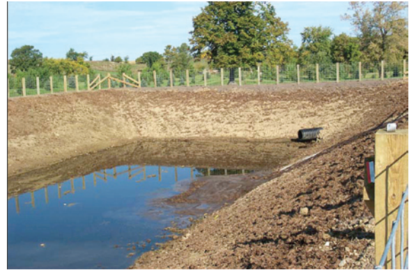
Waste storage facilities at livestock operations help reduce nutrient runoff to the lakes. Project partners installed and improved 50 storage facilities.
