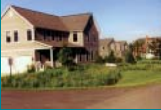
Bioretention with Native Vegetation Prairie Crossing Grayslake, IL
