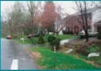
Grassed Swale and Narrow Street Montgomery County, MD
