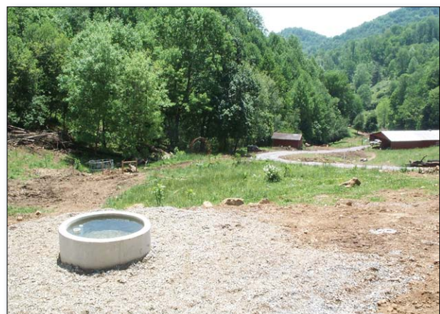
Figure 2. This alternative water source allows livestock to drink without entering Little Ivy Creek.
