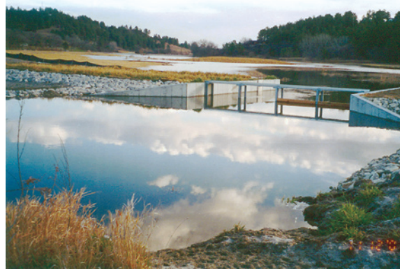
The hydro-suction sediment removal system lies directly beneath the walkbridge shown here.
