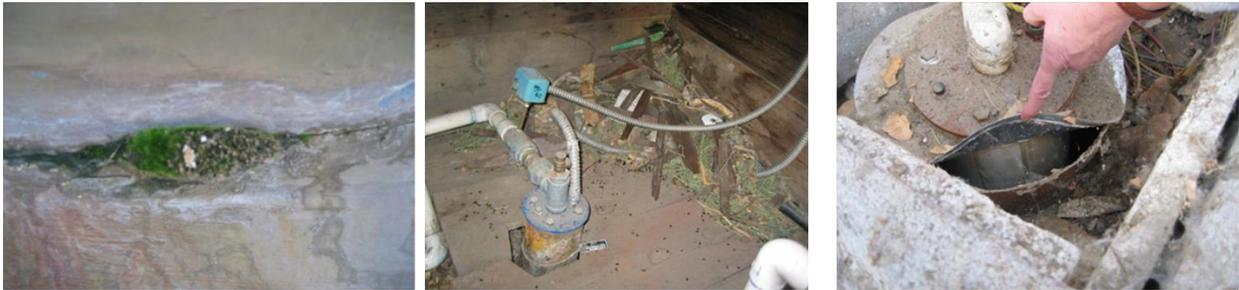
Cracks on a storage tank    Rat droppings around the wellhead    Seal on wellhead not watertight
