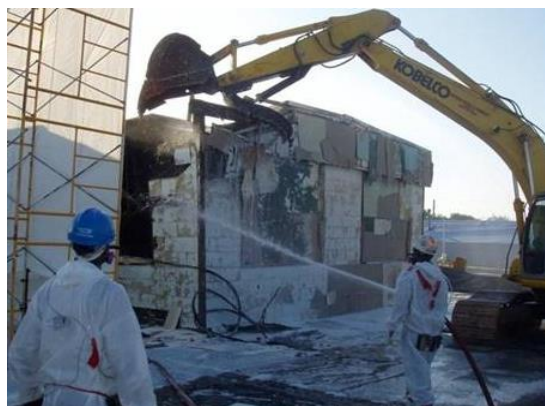
Demolition and wetting of an Alternative Asbestos Control Method building. (EPA photo)
