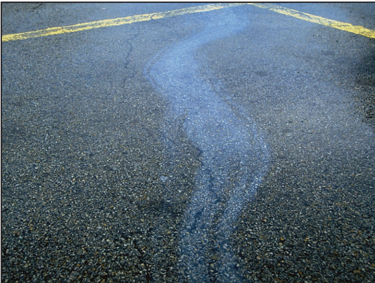
Figure 15. Example of a sheen indicating the presence of oil or other hydrocarbons.
