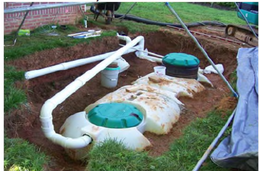
Residential Cistern Project - Installation
