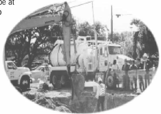
Cleanup in progress on a former industrial site in Clearwater, Florida.
