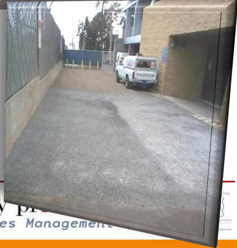
Permeable Alleys (pervious concrete, gravelpave)
