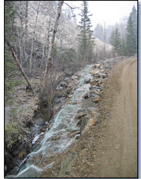
Figure 2. Photo of the project site taken immediately after WDEQ and USFS realigned the road and established a wider buffer area. A white mesh placed on the new riparian area will help hold the soil until vegetation can become established.
