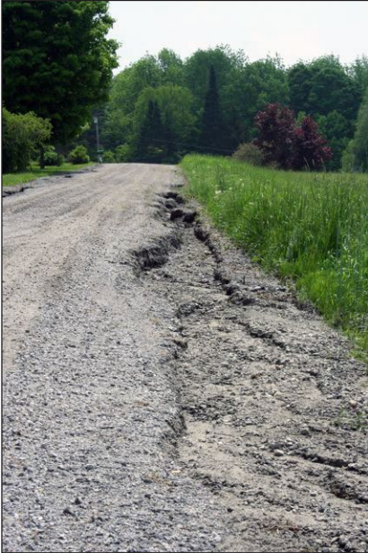
Unpaved roads, such as this one in the town of Plainfield, Vermont, will soon fall under a state general permit. The municipality will be required to ensure the road complies with performance standards or will need to retrofit it with best management practices to prevent erosion. Photo by the Central Vermont Regional Planning Commission.
