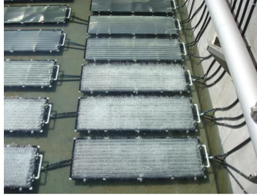
Figure 5-7: Ultra-fine Pore Membrane Aeration Panel
