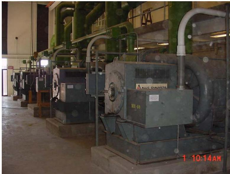
**Figure 3: Multi-stage Centrifugal Blowers - GBMSD - De Pere Wastewater Treatment Facility**
