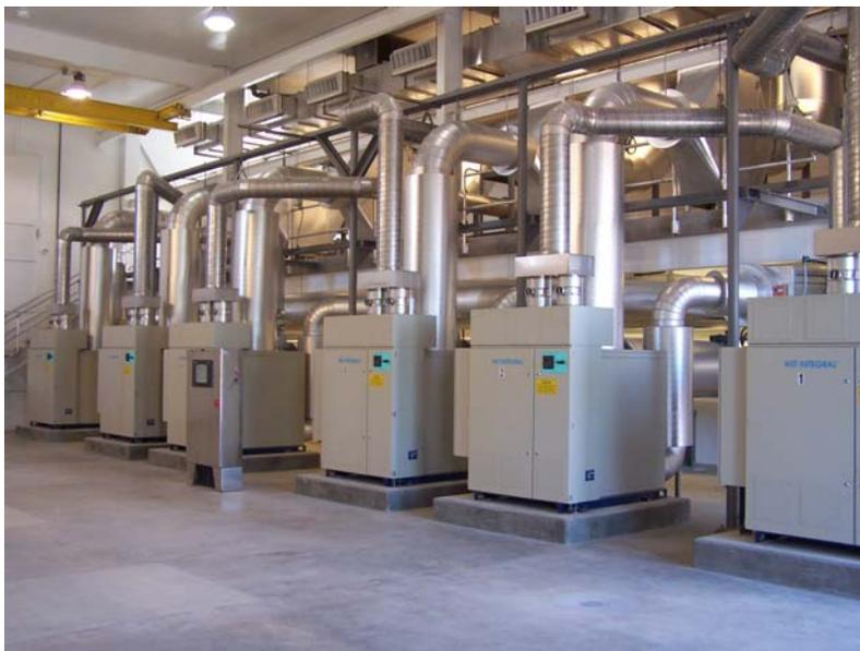
**Figure 4: Magnetic Bearing Turbo Blowers - GBMSD - De Pere Wastewater Treatment Facility**
