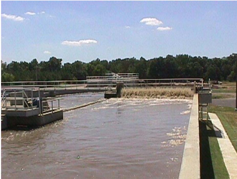
**Figure 2: Oxidation Ditch/Aeration Rotor at the City of Bartlett WWTP #1**
