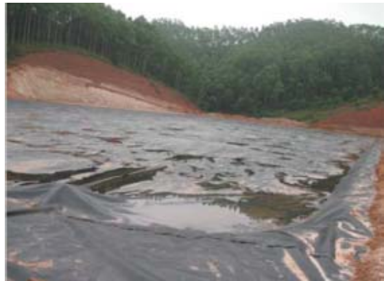
Covered lagoon transferred from GMI demonstration project in Hunan Province
