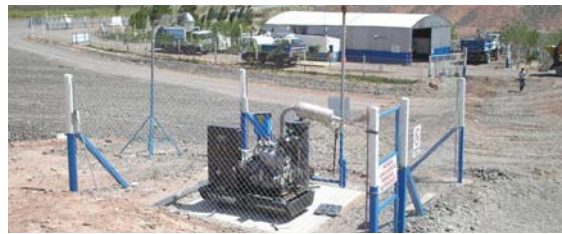
Neuquen Landfill methane collection, burning, and power generation plant
