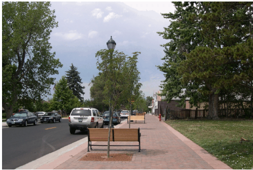
Historic 73 rd Avenue Reconstruction Completed
