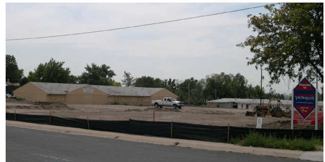
Harris Townhome Project Breaks Ground
