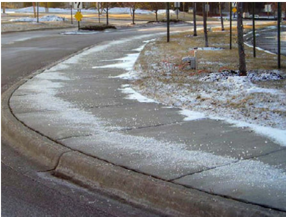
Too much salt was applied to this sidewalk in the City of Plymouth, Minnesota.
