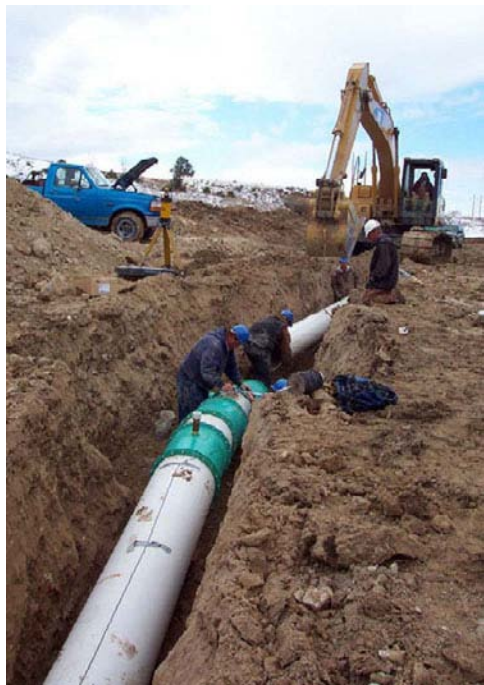
Lateral/Ditch Piping in the Uncompahgre Valley benefits both salinity and selenium reduction. Photo by Mike Baker, Bureau of Reclamation.
