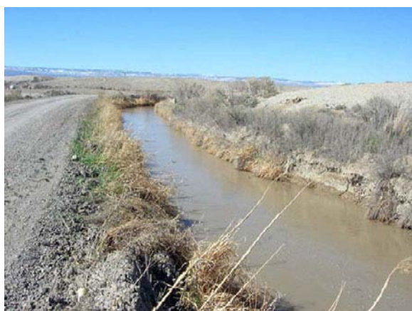
Selig Canal, an earthen canal system proposed for lining in 2007 is located in a high selenium and salinity loading area of the Uncompahgre Valley.
