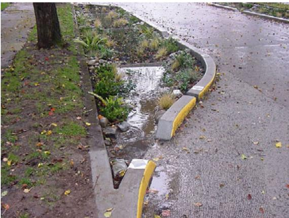
Figure 5. Water flows into the Siskiyou Street curb extension during a rainstorm.
