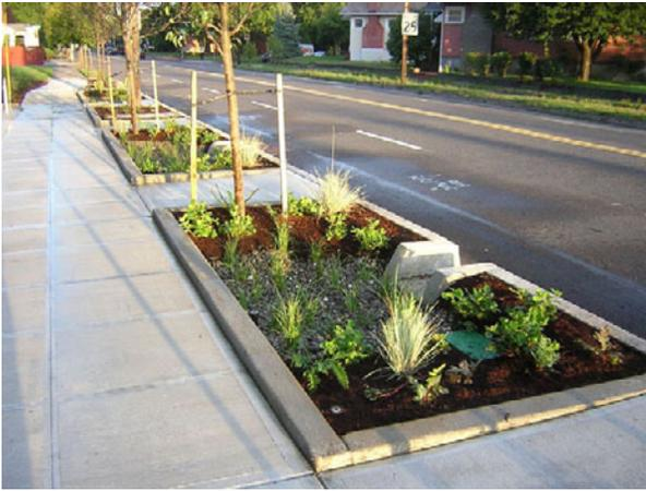
**Figure 7.** These stormwater planters at a shopping area use all available space between the sidewalk and the street for stormwater control.
