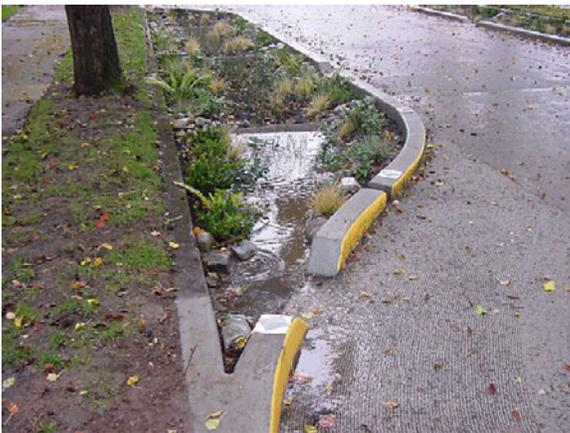
Figure 5. Water flows into the Siskiyou Street curb extension during a rainstorm.
