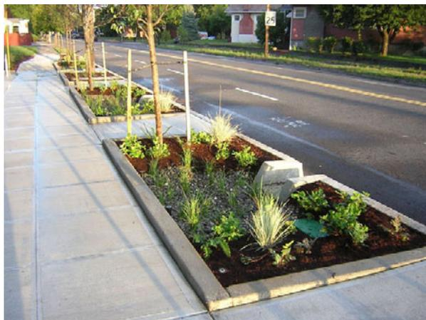
**Figure 7.** These stormwater planters at a shopping area use all available space between the sidewalk and the street for stormwater control.
