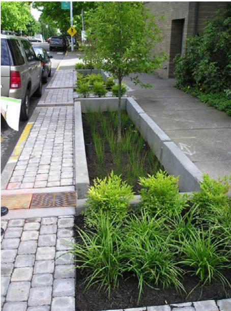
**Figure 8.** Another of the City's stormwater planter systems, installed next to a parking lane, includes a path of pervious block pavers for pedestrian access.
