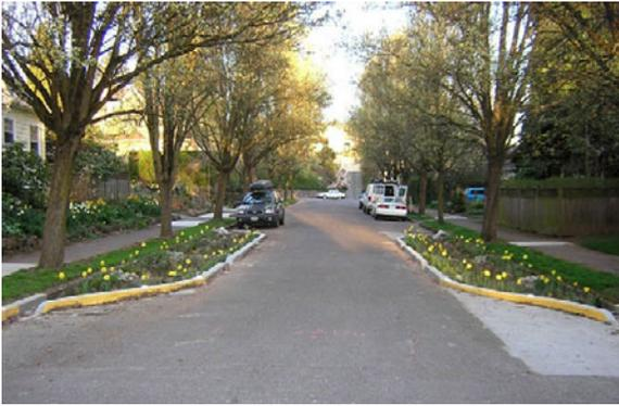
Figure 4. The landscaped curb extensions on Siskiyou Street improve aesthetics, calm traffic, and capture and infiltrate runoff from the street.
