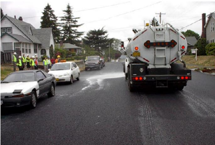
**Figure 10.** Water sprayed from a truck quickly infiltrates through the new curb-to-curb pervious asphalt section of North Gay Avenue.
