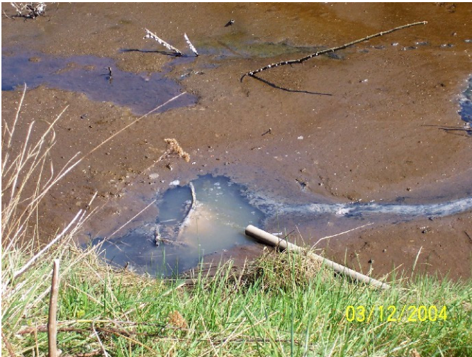
Certified inspectors can spot signs of failing septic systems, such as ponding on the surface, and can work with homeowners to address the problems.
