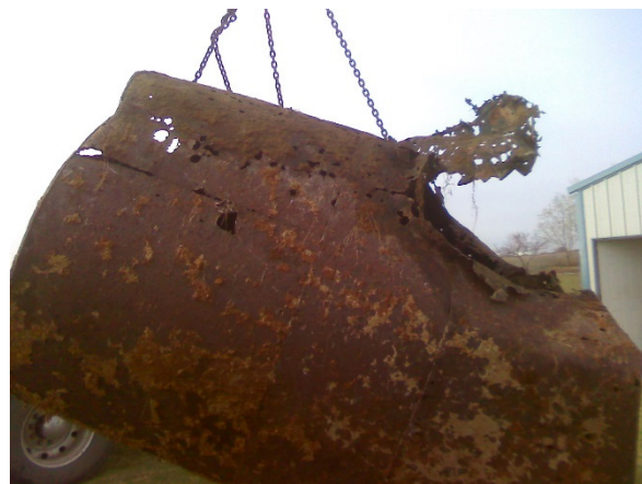
This septic tank failed and needed to be replaced. Oregon's push to increase awareness of the need for septic tanks inspections will help ensure proper septic tank operation.
