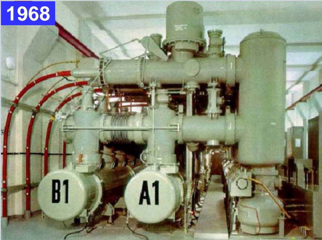
Since more than 40 years in service Berlin, UW Wittenau, Vattenfall Europe, 123 kV, 31.5 kA
