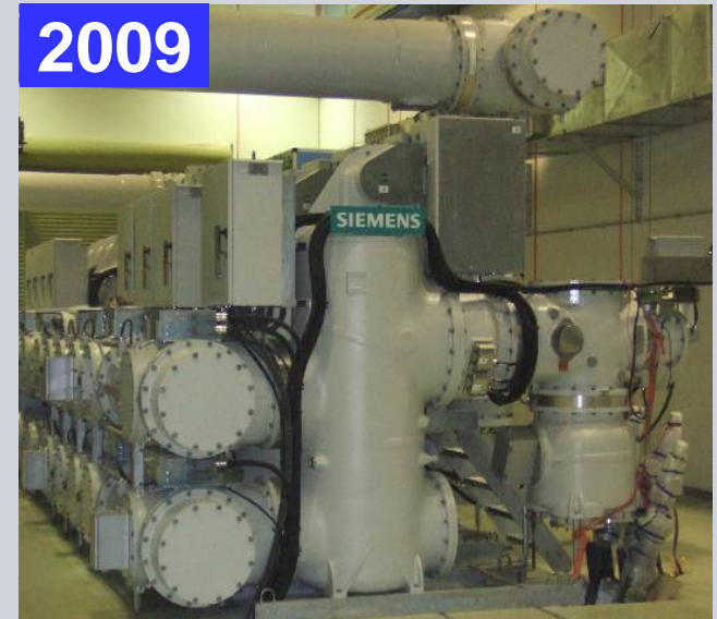
State-of-the-art 145 kV, 40kA GIS
