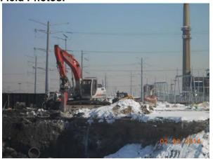
Photo 1: Excavator breaking frost layer in Area 5S.
