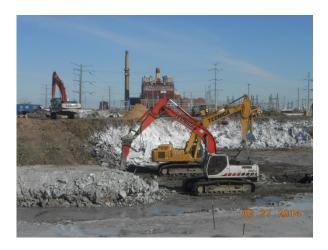
Photo 1: Breaking down concrete structures in Area
