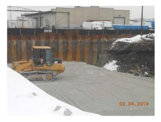
Photo 3: Backfilling in the northwest corner of Area 5S and 6E.
