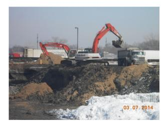
Photo 2: Loading trucks from eastern wall of Area
