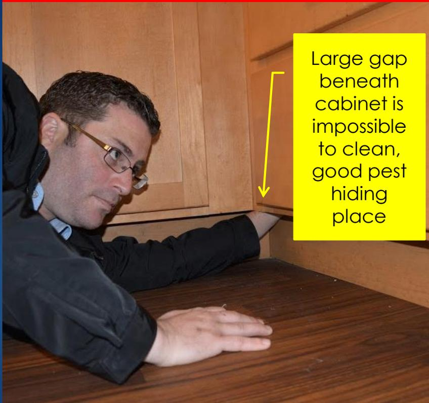
Large gap beneath cabinet is impossible to clean, good pest hiding place
