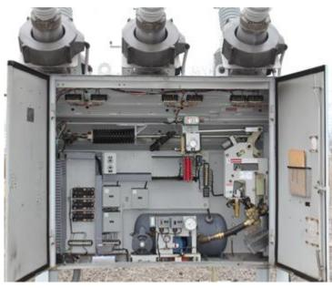
Butler, PA 38 kV, 1200 A 6.8 kg SF<sub>6</sub> ~0.17 m<sup>3</sup> 75 psig at 21.1 °C The advanced sensor has passed type tests, cold test, and is currently completing one-year field testing
