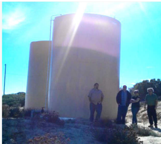
Final installation of two 20,000-gallon water storage tanks
