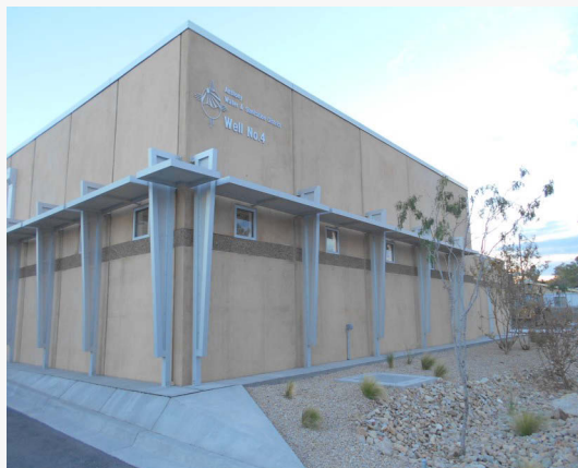
New well station in Anthony, N.M.
