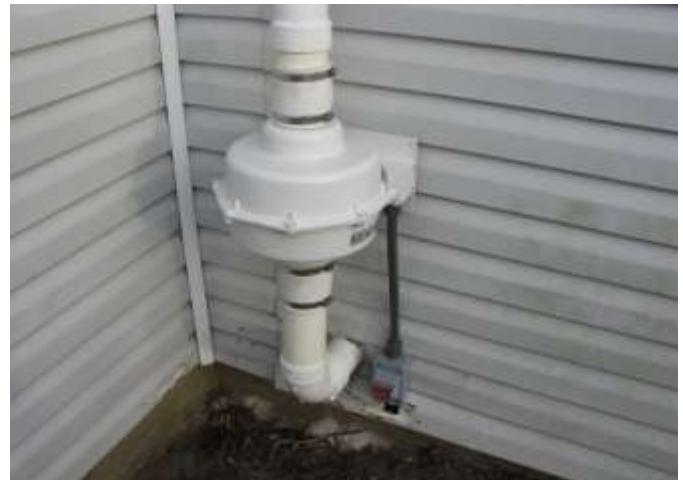
This fan outside the house is part of a vapor abatement system.
