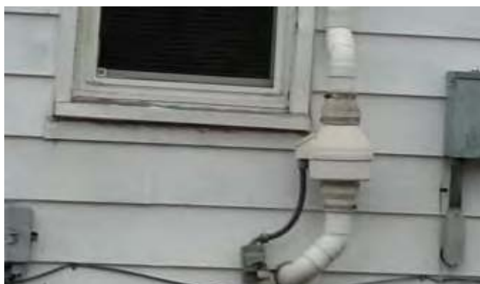
This photograph shows a VAS installed on the outside of this house.
