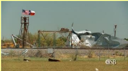
Damaged tanks at the West Fertilizer site. (U.S. Chemical Safety and Hazard Investigation Board (CSB) photos)
