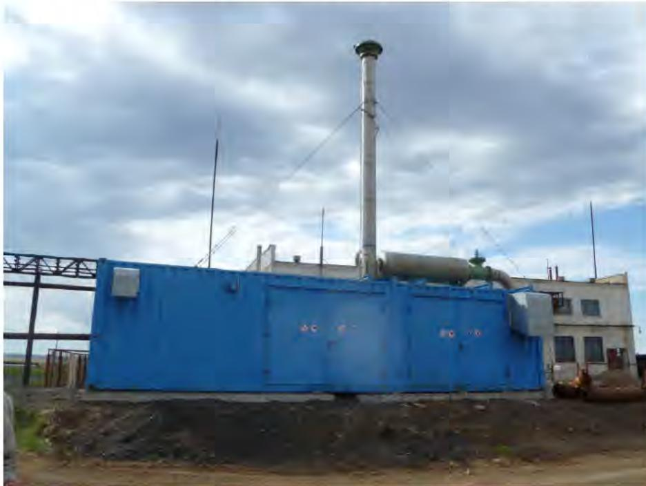
These PD blower stations are automatically controlled and require very little modification to enable safe utilization of drained gas. The PD blower pumps can be configured to vary the speed to maintain a variety of parameters such as methane concentration, vacuum, or back pressure.
