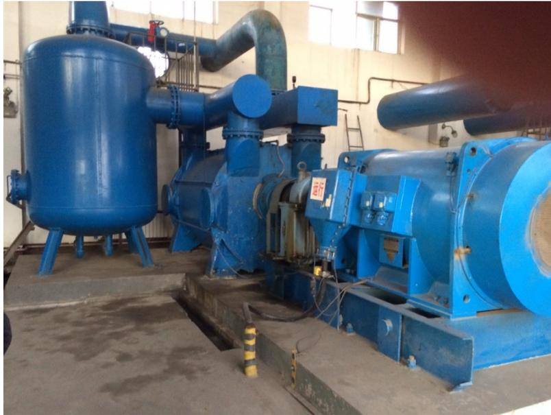
**Figure 4-2: Vacuum pump at the Pingshang Mine**
