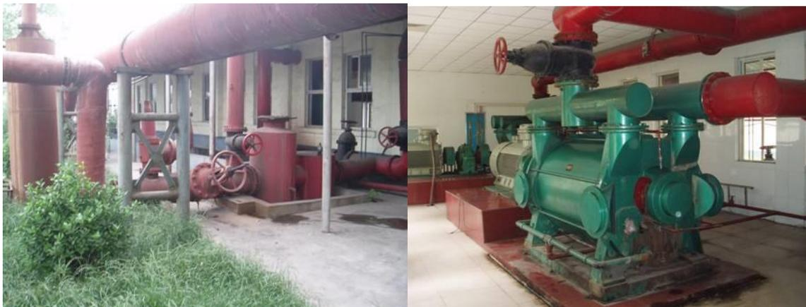
**Exhibit 1-9: Surface Gas Collection and Water Separation (on left), Vacuum Pump (on right)**
