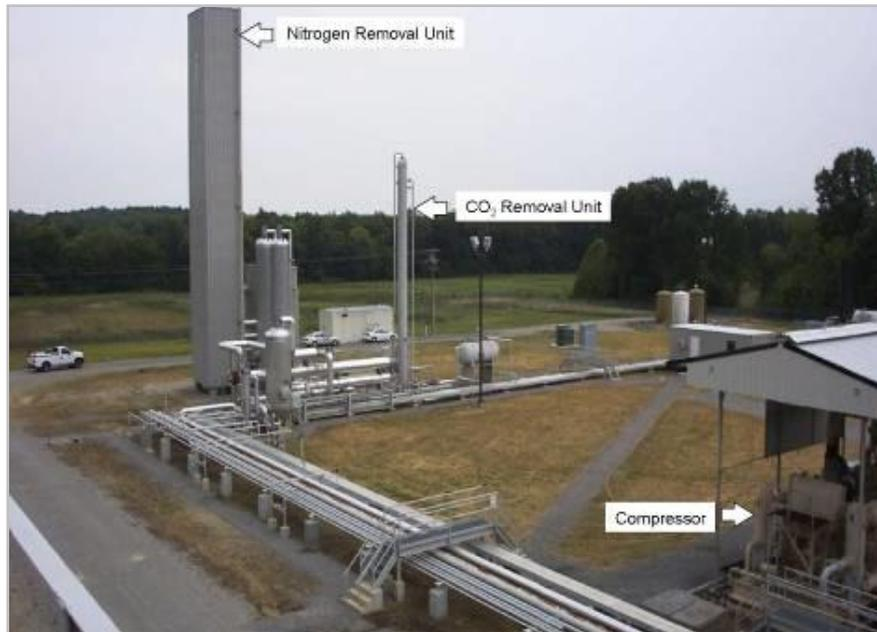
**Exhibit 5-9 CO<sub>2</sub> Unit, Nitrogen Rejection Unit and Compressor**
