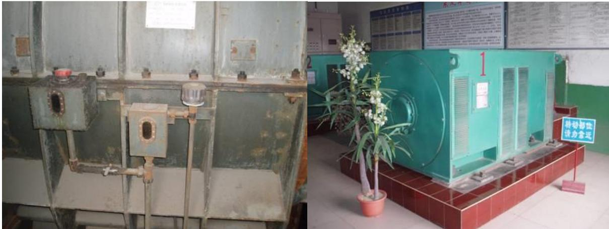
**Exhibit 1-19: Fan Housing with Sensors (left) and Electric Motor (right).**
