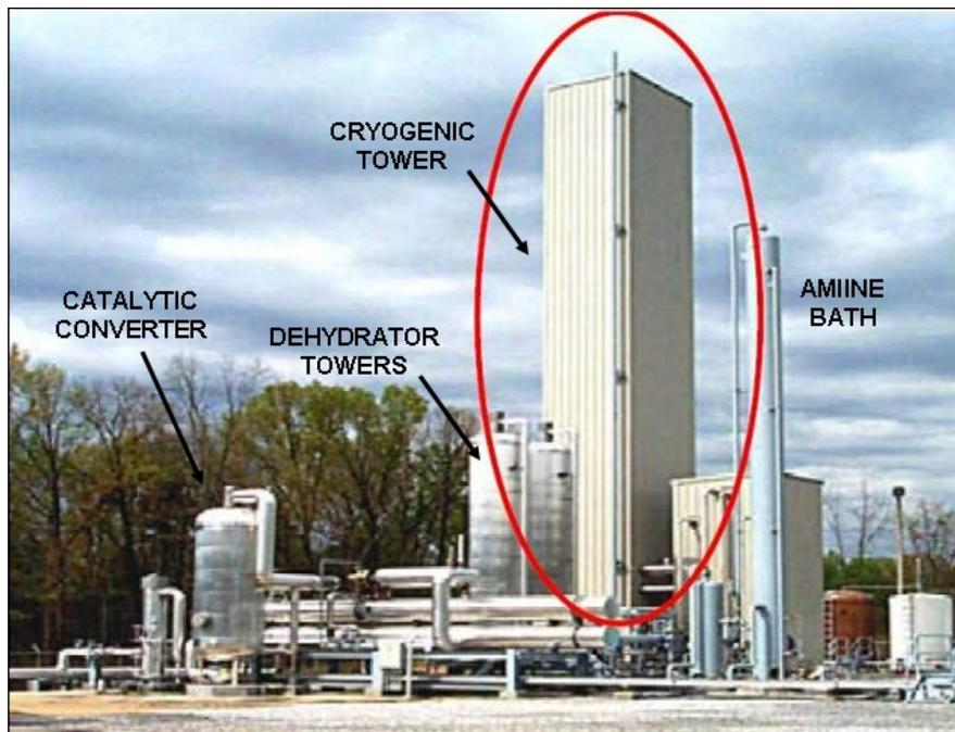
**Figure 5-7: Cryogenic Gas Processing Plant**
