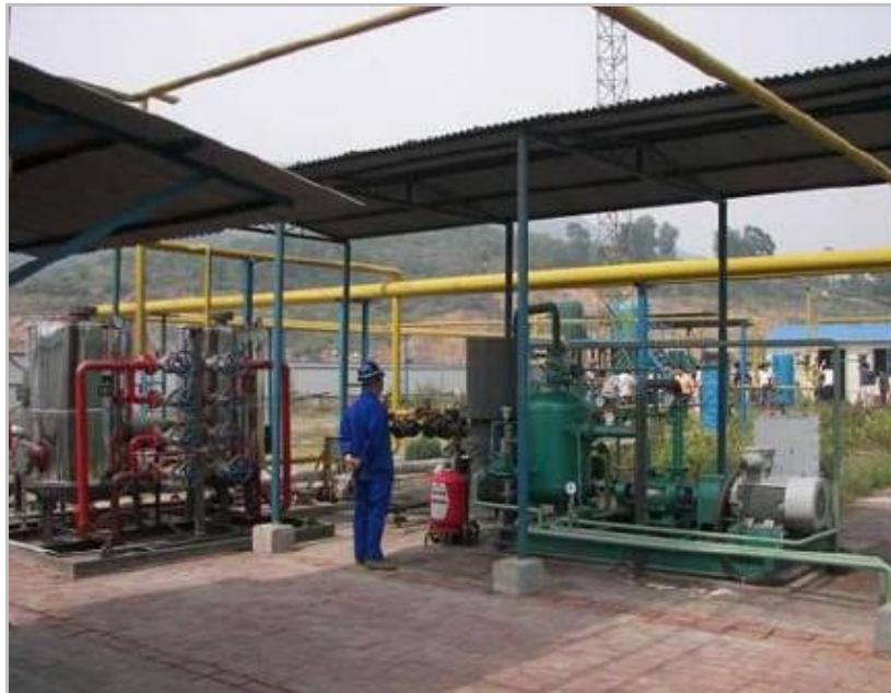
**Figure 5-8: Test-Scale CMM-to-LNG Plant, Shigang mine, Shanxi Province**
