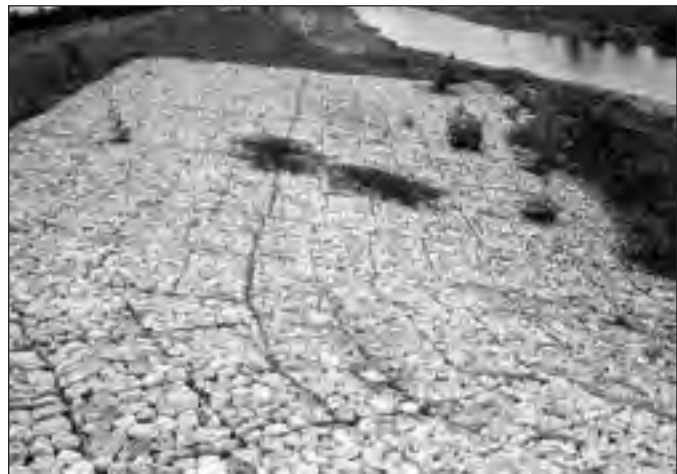
Riprap (rock cover) reduces stream channel erosion (left) and gabions (crushed rock encased in wire mesh) help stabilize erodible slopes (right).
