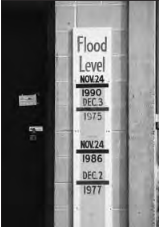
Knowing the behavior of waters at their peak flood level is important for determining whether waste will wash out.
