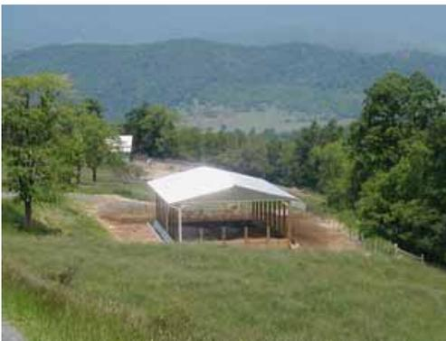
Animal feeding area after installation of waste storage facility, runoff control system, stream fencing, clean water diversion, paved feeding area, livestock watering facility, stabilized access road, and critical area planting.
