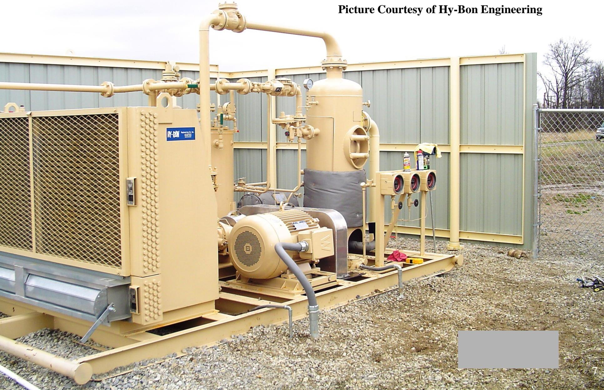
**Rotary Screw compressors were used due to the wet nature of this gas stream. Filters are used before the skid to remove iron sulfide, then a scrubber vessel and automated liquid transfer system on skid to handle the liquids which are common in this application.**
