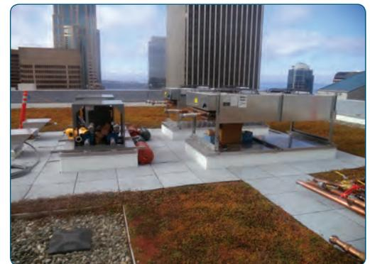
Above: The new cooling system takes air from the outside and filters it into the server/network room at much lower cost than the previous air conditioning units.
