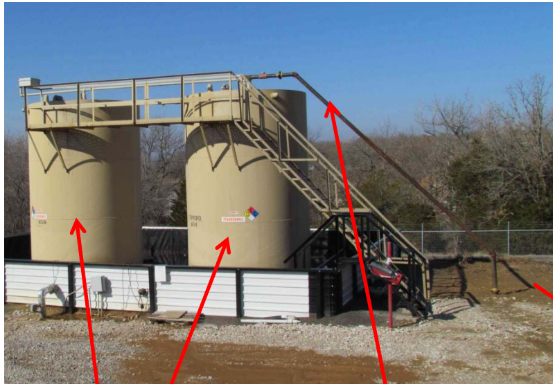
Boil-off gas collection pipe
