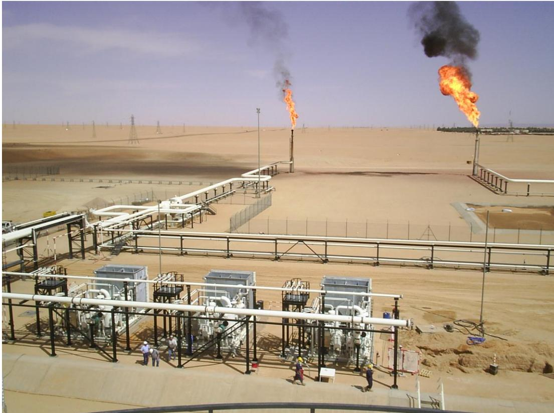
Picture of the flares at NC-115 after the VRU's were installed. Units capturing 4 MMscfd (Four million standard cubic feet per day) of previously flared or vented natural gas streams.
