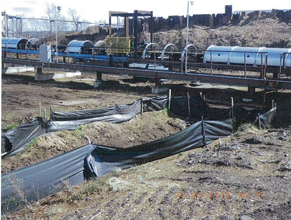
Photo IMGP9049: Silt fencing around the ditch at the north end of the construction area with identifiable rips and missing segments. Direction: Facing northeast.
