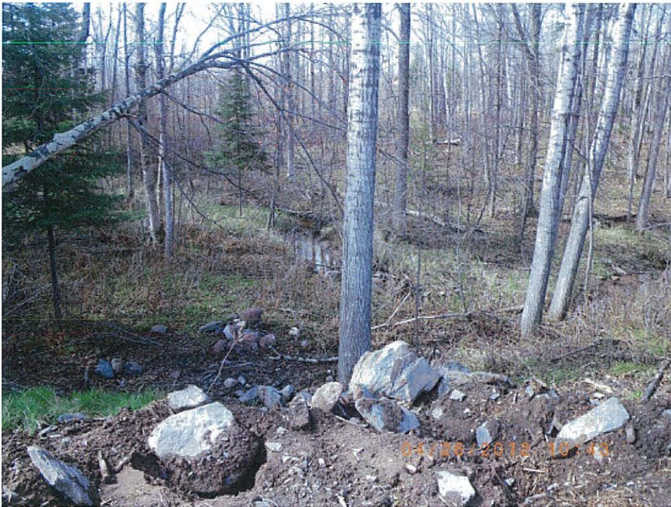
Photo IMGP9054: Soil and rock that was piled along the western side of the construction with identifiable runoff pathways leading towards the stream. Direction: Facing southwest.
