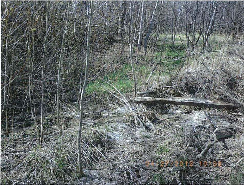
Photo IMGP9095: Vegetated area of the ditch originating at the northwest corner of the wood room building. Direction: Facing west.
