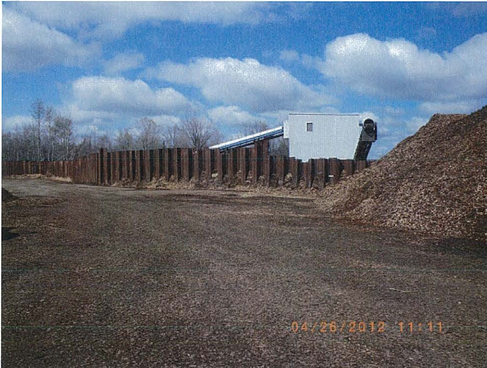
Photo IMGP9066: Pilings along the north side of the access road surrounding the wood chip pile. Direction: Facing northwest.
