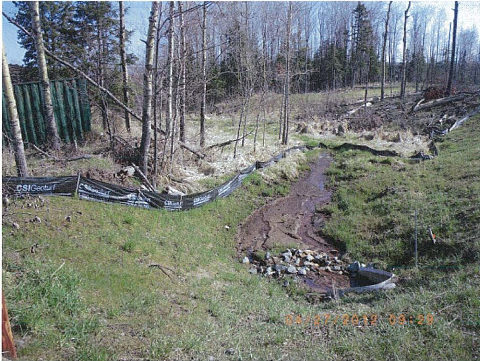
Photo IMGP9078: Culvert from under U.S. Highway 41 flowing onto the FAF. Direction: Facing northeast.
