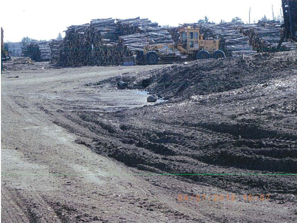
Photo IMG9092: Culvert from the Verso wood storage area. Direction: Facing east.
