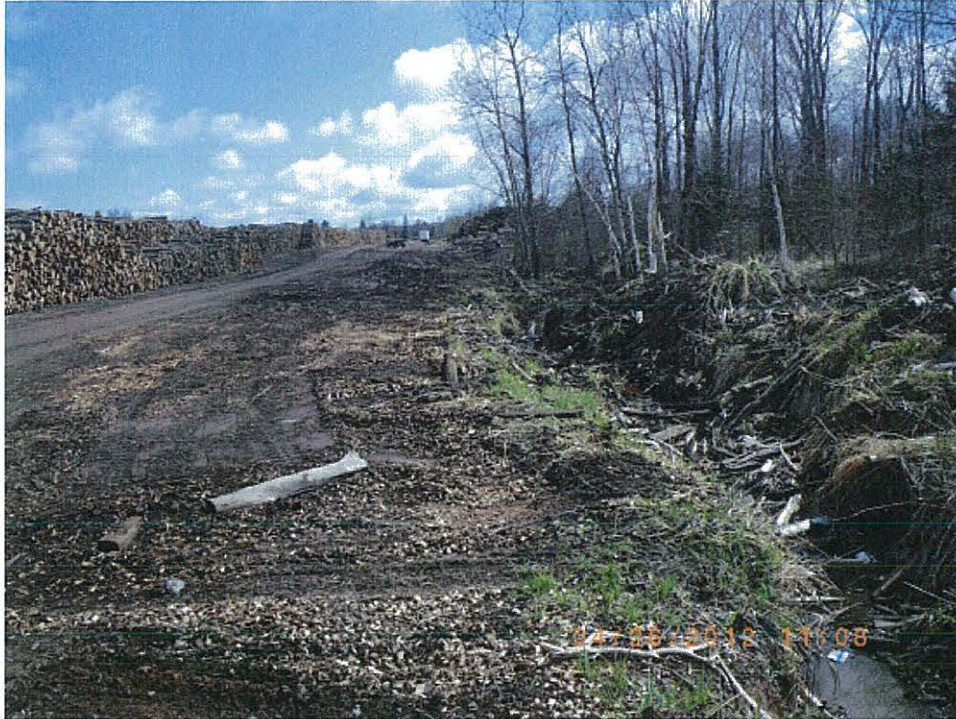
Photo IMGP9063: Ditch at the north end of the PCP aggregate with water and debris present. Direction: Facing east.
