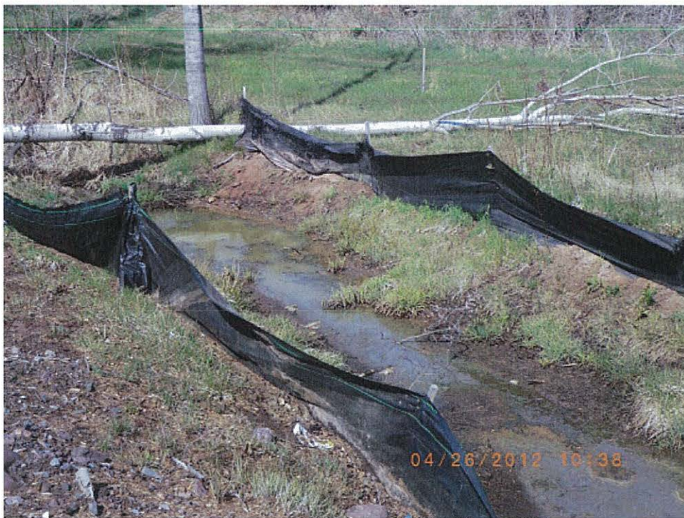
Photo IMGP9050: Silt fencing along the ditch at the north end of the construction area. Direction: Facing northwest.
