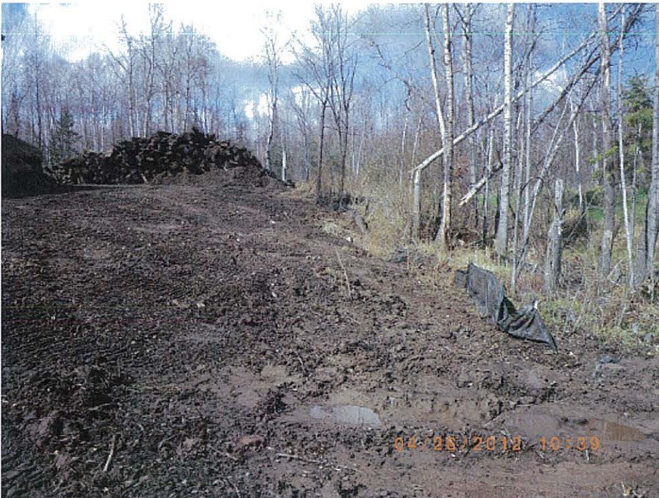
Photo IMGP9052: Loose soil located at the construction area along the west side of the processed railroad tie storage building. Direction: Facing west.
