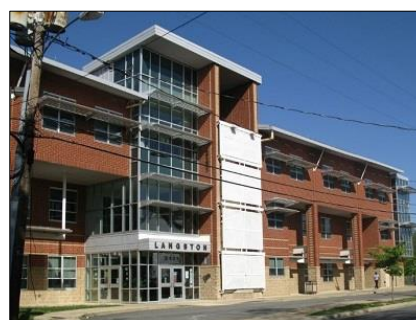
Figure 28: The 11,000-gallon cistern behind the white screen at the Langston-Brown Community Center in Arlington, Virginia, stores rainwater to reuse for onsite irrigation.
