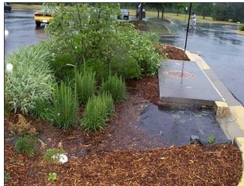
Figure 30: Existing developments can retrofit parking lots to add green infrastructure elements in medians and perimeter landscape areas.
