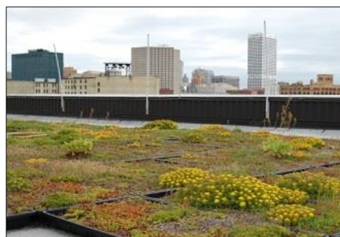
Figure 29: Lightweight and easy-to-maintain green roofs can be added to existing roofs.
