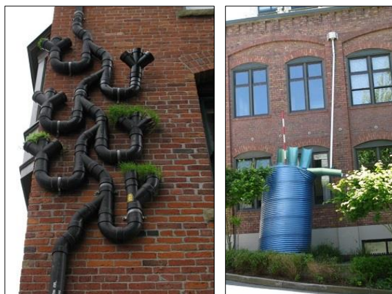
Figure 21: Stormwater-capture devices, such as these in Seattle, can be artistic as well as functional.
