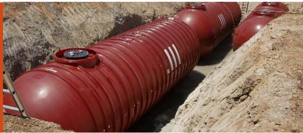
Secondary containment uses a barrier, an outer wall, or a liner around the UST or piping to provide secondary containment. Tanks can also be equipped with inner bladders that provide secondary containment.
