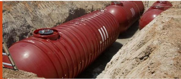
Manual tank gauging requires keeping the tank undisturbed for at least 36-58 hours each week, during which the contents of the tank are measured twice at the beginning and twice at the end of the test period. At the end of each week, you compare the results to the standards shown on page 25 to see if your tank is leaking.
