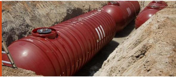
Vapor monitoring measures either product vapors in the soil around the UST, referred to as passive monitoring, or special tracer chemicals added to the UST, referred to as active monitoring.
