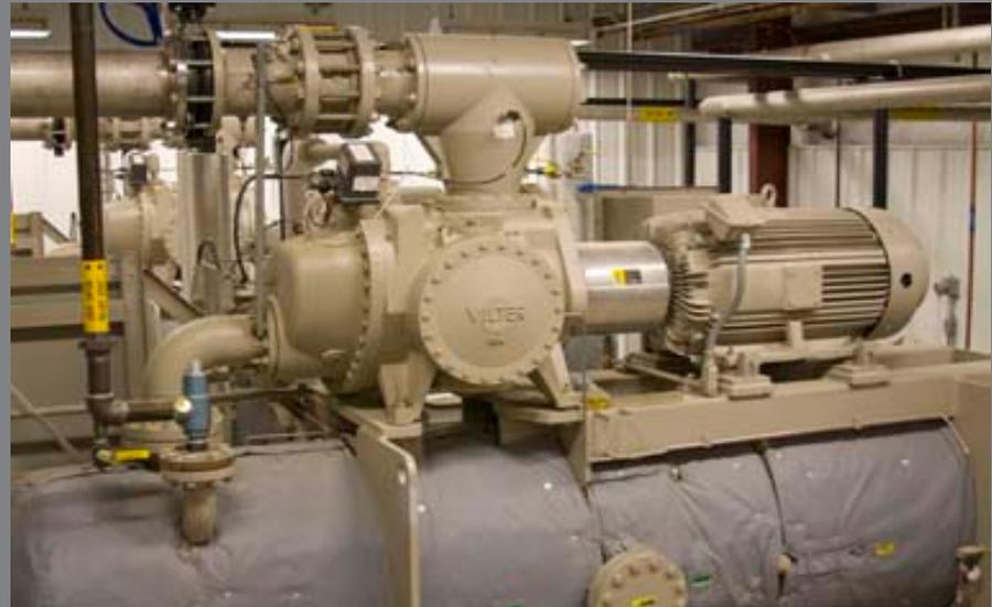
LFG is Compressed and Chilled to Drop Out Moisture Prior to Conveyance Through a Three Mile Pipeline to the Engine Generator Building
