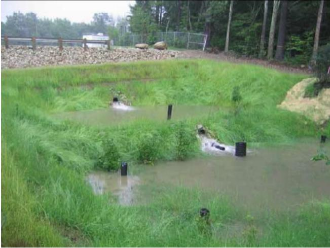
Figure 16. Gravel wetland (Ballestero et al. 2011)
