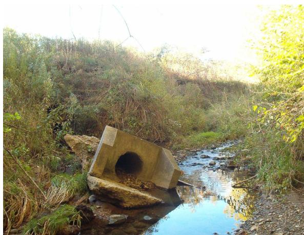
**Figure 5.7 Fallen end section in Glazier Reach**
