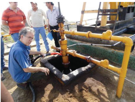
Dr. Alfredo Barriga demonstrates gas leak measurements on an oil well.
